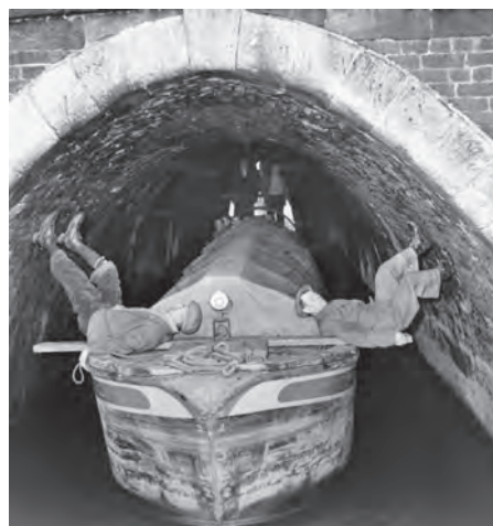
Two 'leggers' in the 500 yard Barnton Tunnel on the Trent and Mersey Canal in 1961
